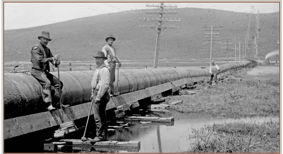
Crystal Springs Pipeline No. 1 after earthquake 1906
