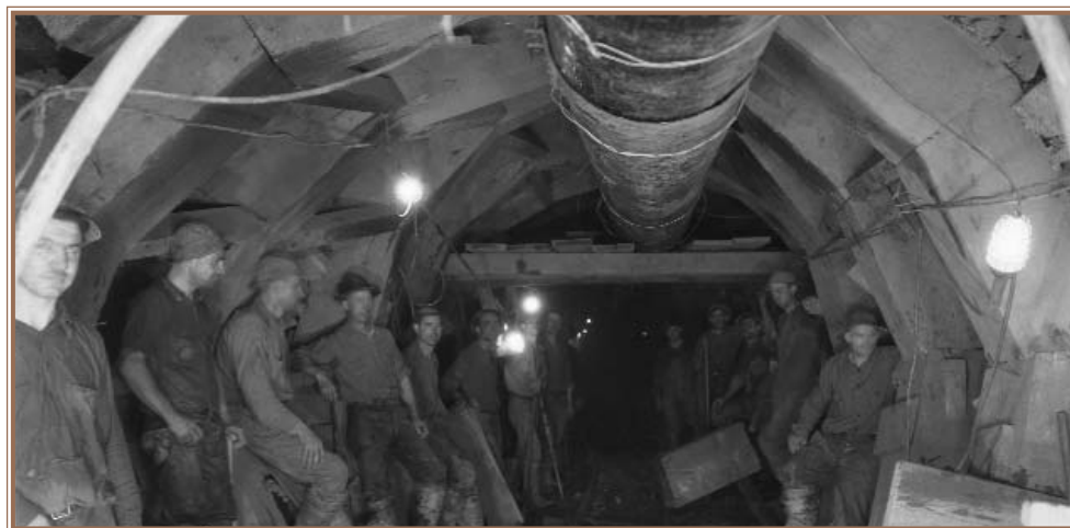
Construction workers in Coast Range Tunnel 1930
