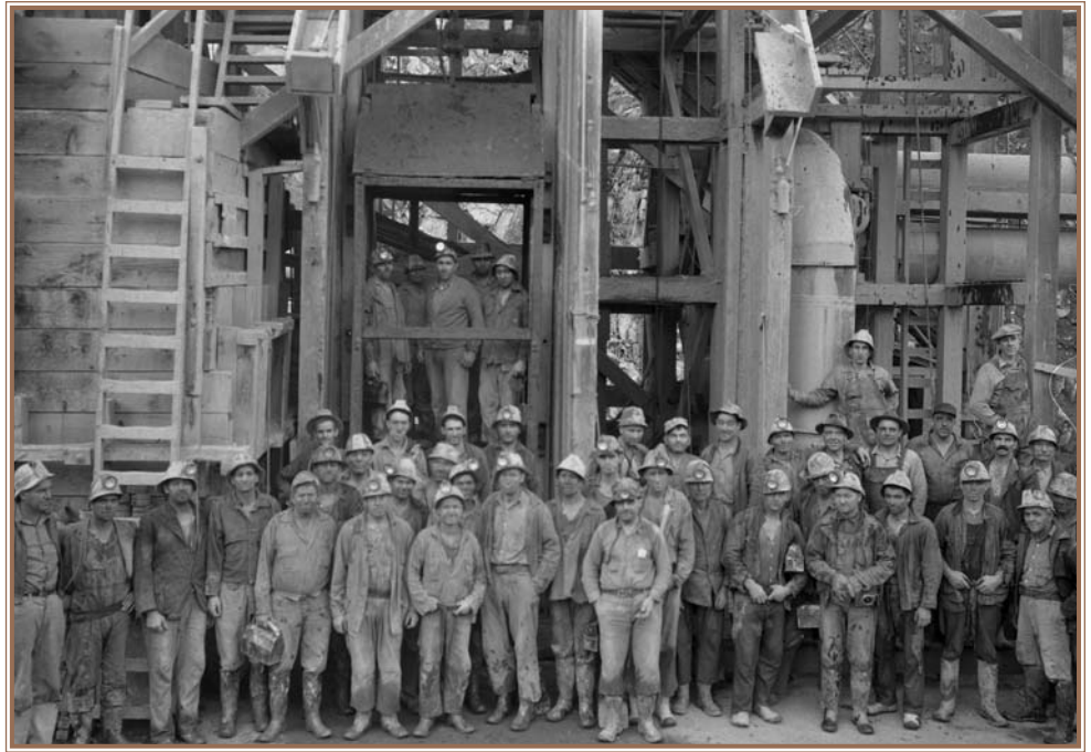
Coast Range Tunnel workers outside Mitchell Shaft 1934
