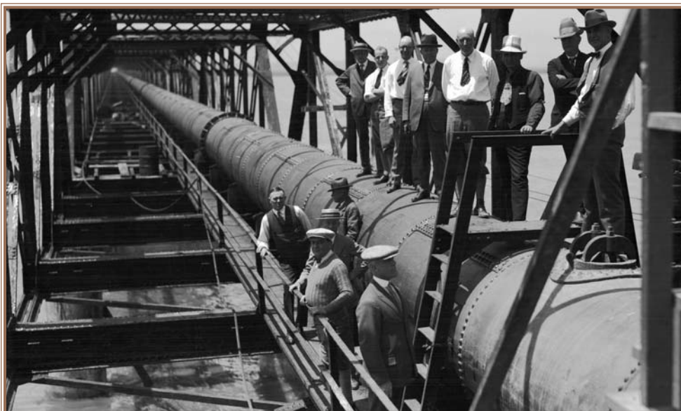
Bay Division Pipeline No. 1 on Trestle Bridge 1925
