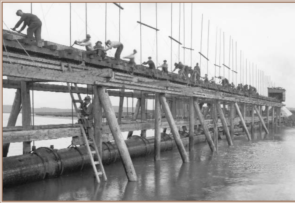
Construction of submarine sections of Bay Crossing Pipeline No. 1 1925
