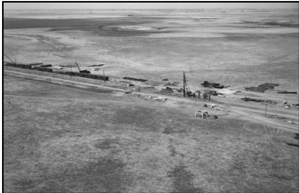
Trestles being rebuilt in 1950s
