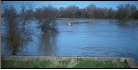
Water flowing over the Fremont Weir
