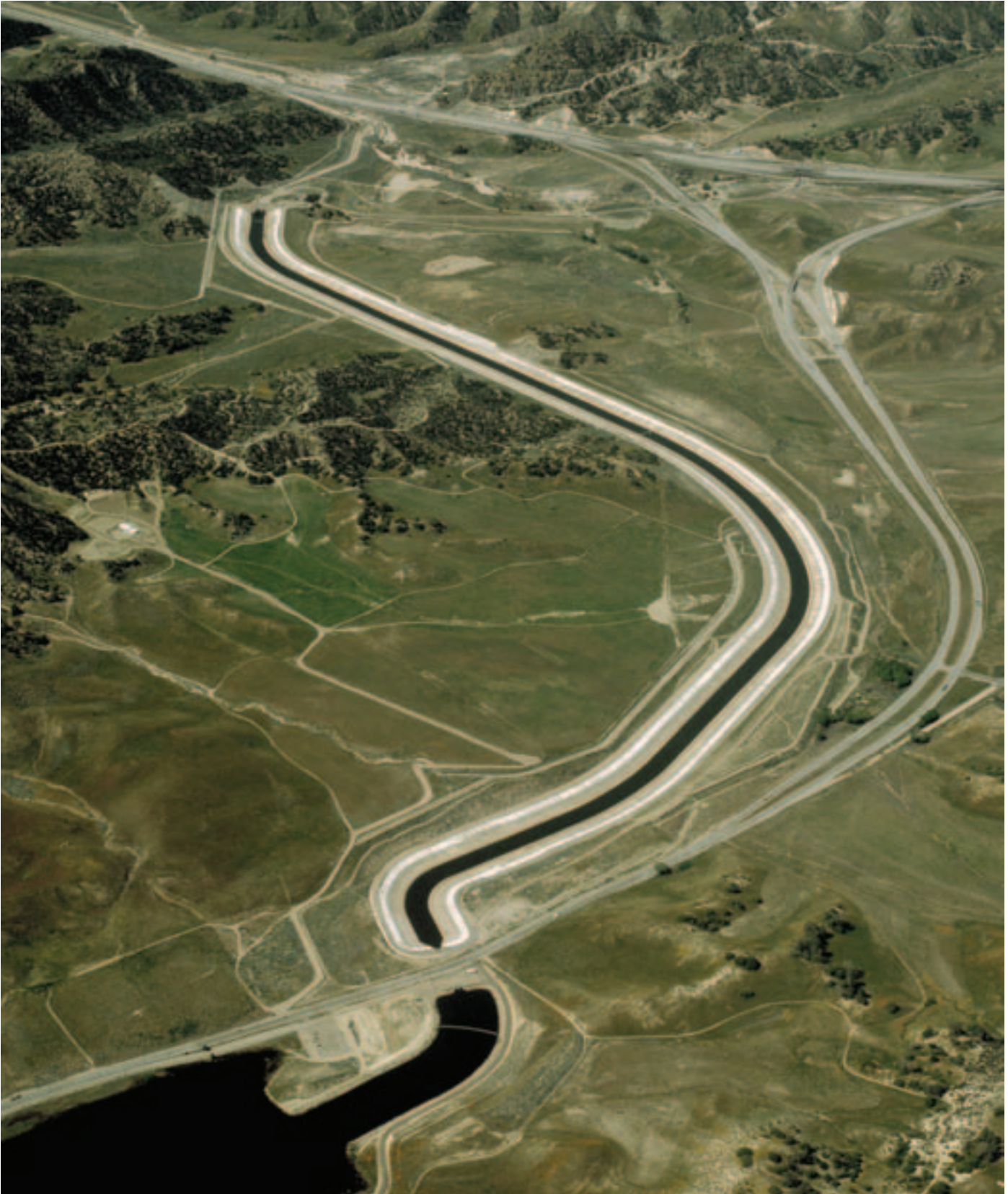
Conveyance infrastructure includes natural watercourses as well as constructed facilities. An overall objective is to balance the operation and maintenance of conveyances to meet the needs of all sectors. (DWR photo)
