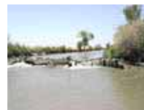
Photo 4-21 Yolo Bypass toe drain—Lisbon Weir /DWR photo
