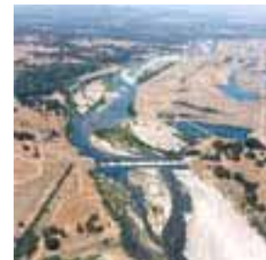
Photo 4-11 Yuba River— Daguerre Point Dam
