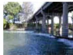
Photo 4-27 Tuolumne River—Dennett Dam (Stanislaus County)/DWR Photo
