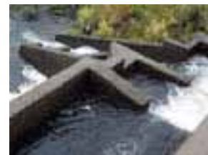
Photo 4-15 Cosumnes River—fish ladder at North Granlees Dam (Retrofitted in 2003)/DFG photo
