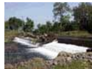
Photo 4-9 Deer Creek—Stanford-Vina Ranch Diversion Dam /Photo
