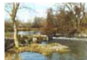
Photo 4-6 Lower Butte Creek Project East-West Weir—Sutter Bypass / DFG Paul Ward photo
