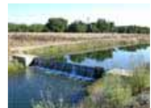
Photo 4-22 Mormon Slough—flashboard dam /DWR photo
