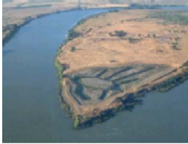
Figure 10. Aerial photograph with superimposed design of Decker Island breached wetland project. The design is similar to Kimball Island project in that it has limited opening to the river and consider length of interior channels. Like Kimball the interior channels of Decker have become clogged with water hyacinth and where the fish community is dominated by non-native species.
