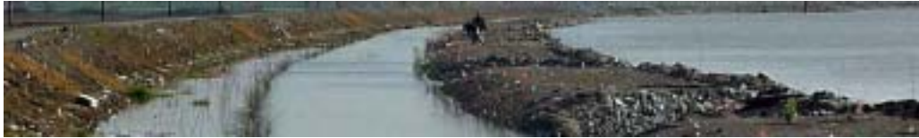
Installing woody vegetation on old levee (March 2000)
