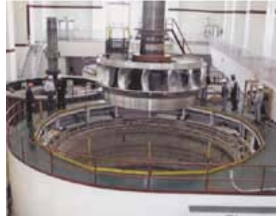
Workers perform upgrades to the turbine at the Shasta Power Plant.
