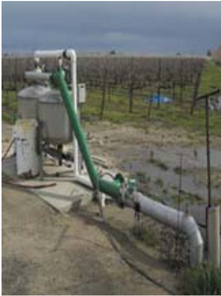
Ground water pumping in the Central Valley
