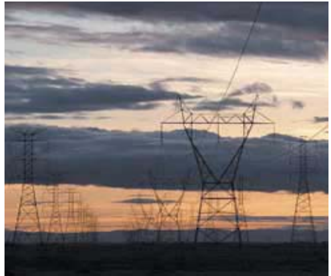
Power lines distribute electricity produced by CVP hydropower generators.
