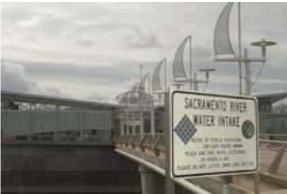
The city of Sacramento's new pumping plant on the Sacramento River.
