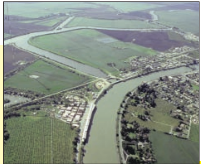
Sacramento River bend, with Delta Cross Channel (at left) flowing into Snodgrass Slough and down toward the Mokelumne River.
